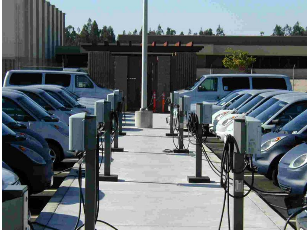
Figure 4. TH!NK city charging infrastructure at Vandenburg Air Force Base.
