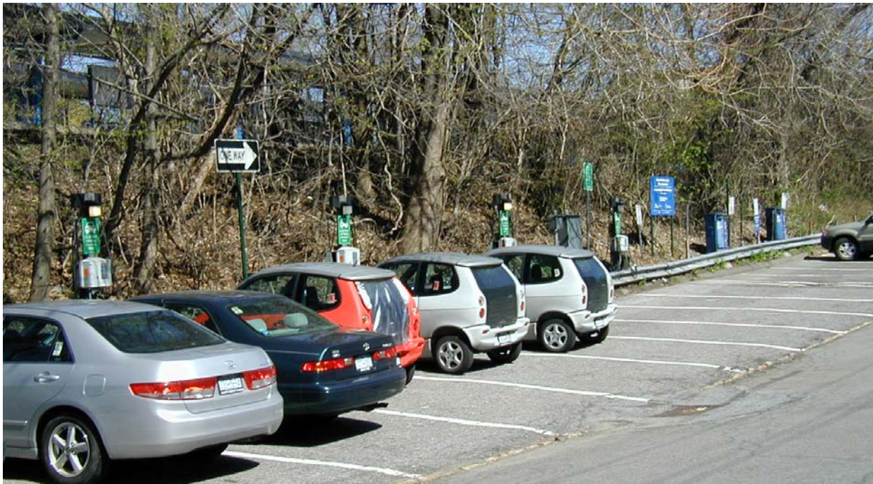
North White Plains, Westchester County— Eight Chargers.
