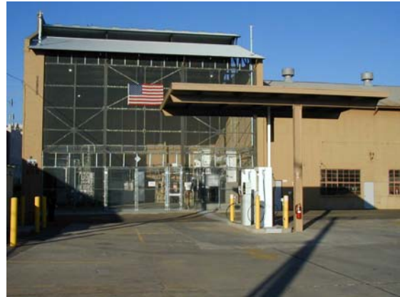
Figure 1. APS Alternative Fuel Pilot Plant and fueling pumps.
