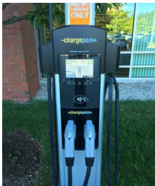
Figure 22. Dual port ChargePoint EVSE at Dunkin Brands headquarters.
