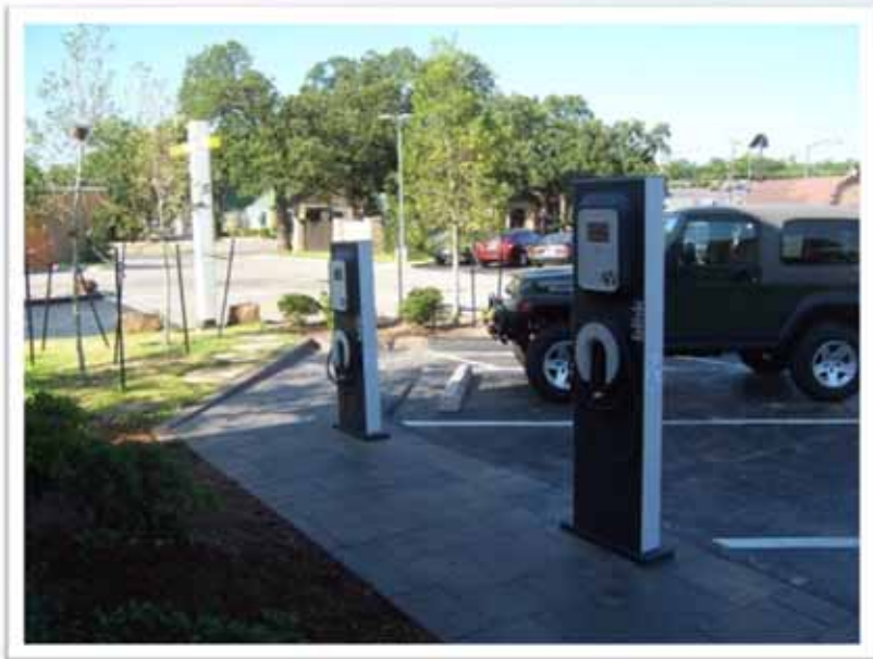
Pedestal EVSE installed on decorative paving ; removal and replacement required for underground conduit
