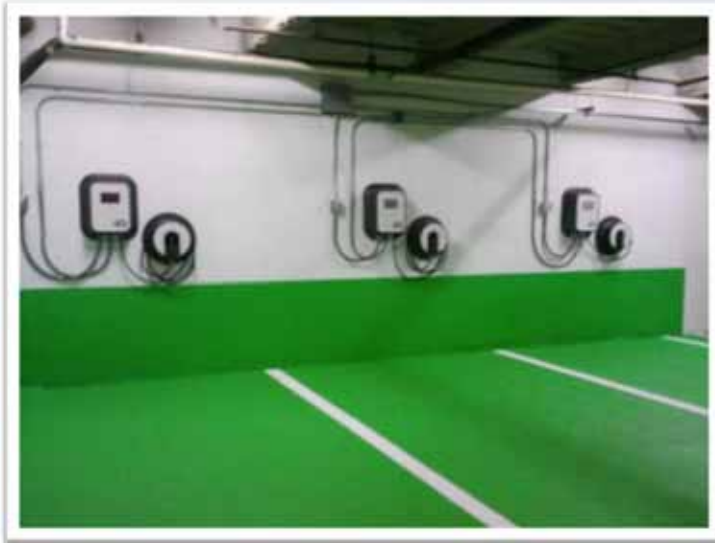
Wall-mounted EVSE installed in parking garage with overhead surface-mounted conduit
