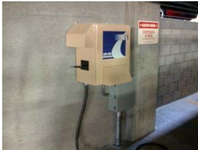
Figure 5. LSV-100 NEV charger in the City of Palm Springs' City Hall parking garage.
