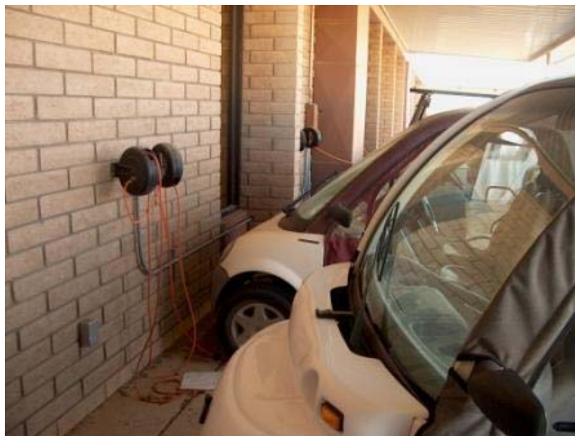
Figure 2. Luke Air Force Base NEV charging outlets.
