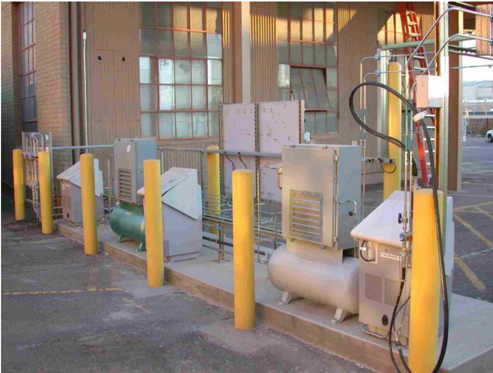
Figure 4. FuelMaker with HCNG mixer.
