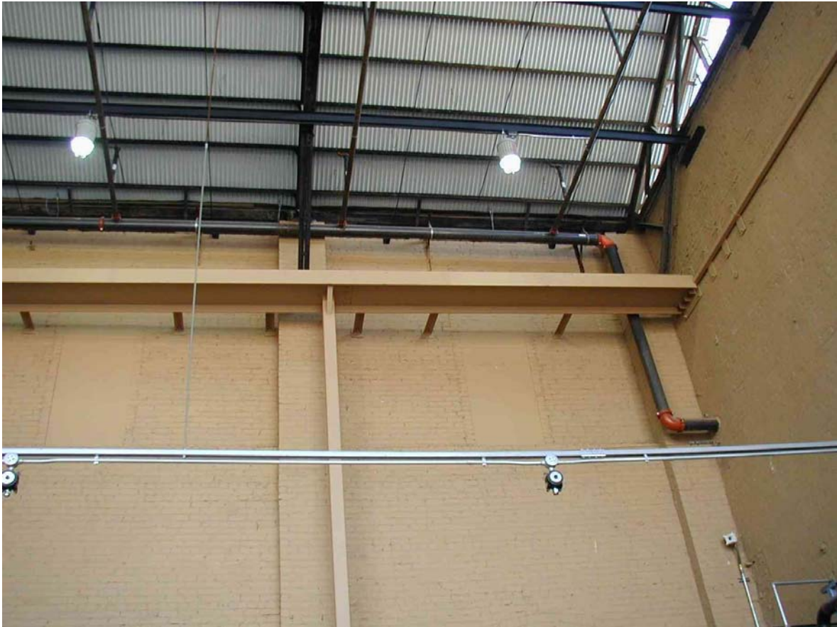
Figure 1.3. Building Reinforcement.
