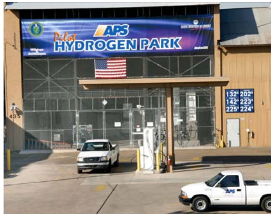
Figure 4-3. Arizona Public Service Alternative Fuel Pilot Plant.
