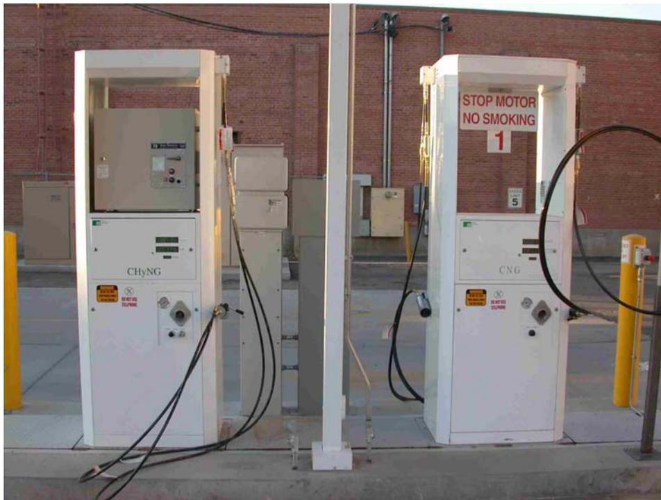
Figure 2. Fueling Technologies Inc. fuel dispensers (CNG and hydrogen/CNG blend fuels).
