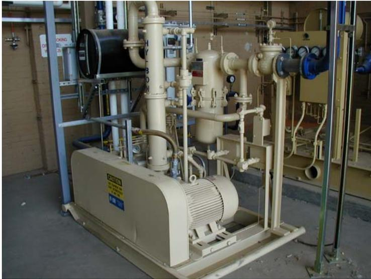
Figure 3.1. Hy-Bon - CNG boost compressor.
