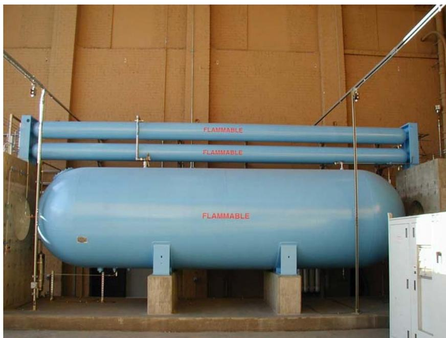
Figure 2.3. Hydrogen low-pressure storage vessel is the large tank on the bottom and the two high-pressure storage vessels are on top.
