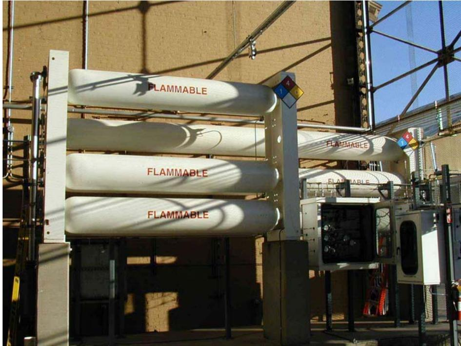
Figure 3.3. CNG storage tanks. The top tank is the high-pressure tank and the two lower tanks are the medium-pressure tanks in the near rack. The three low-pressure tanks are in the far rack.
