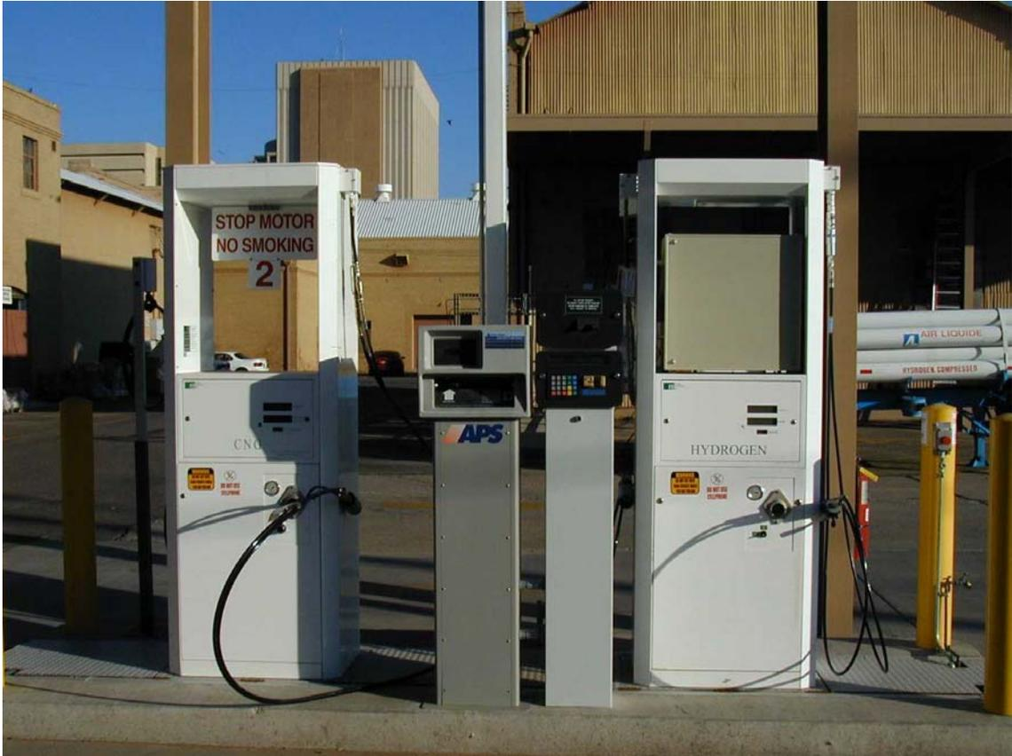
Figure 2.4. CNG only dispenser and hydrogen and CNG/hydrogen blend dispenser.
