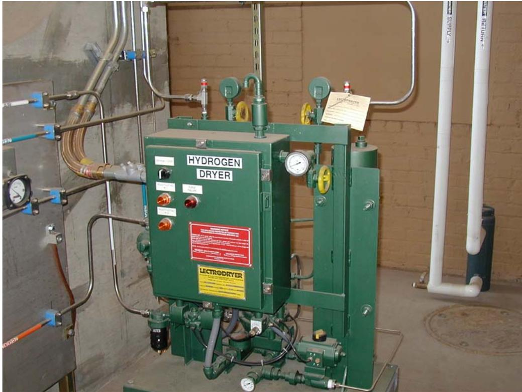
Figure 2.2. Lectrodryer hydrogen dryer.
