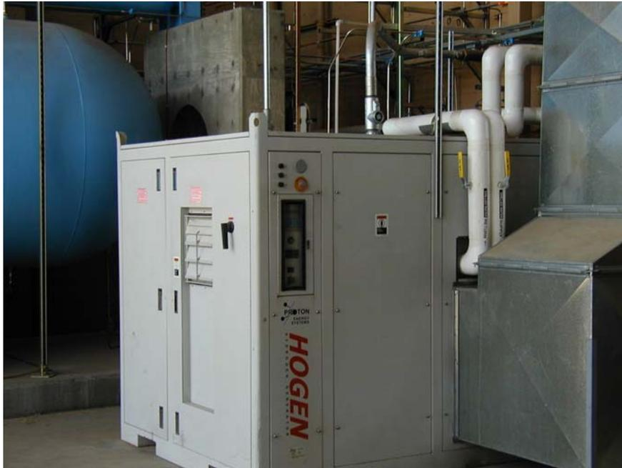
Figure 2-1. HOGEN 300 proton exchange system.
