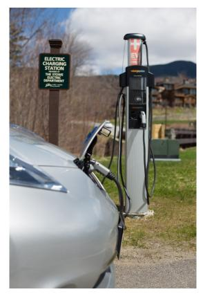
Figure 15. ChargePoint Level 2 EVSE in Stowe.
