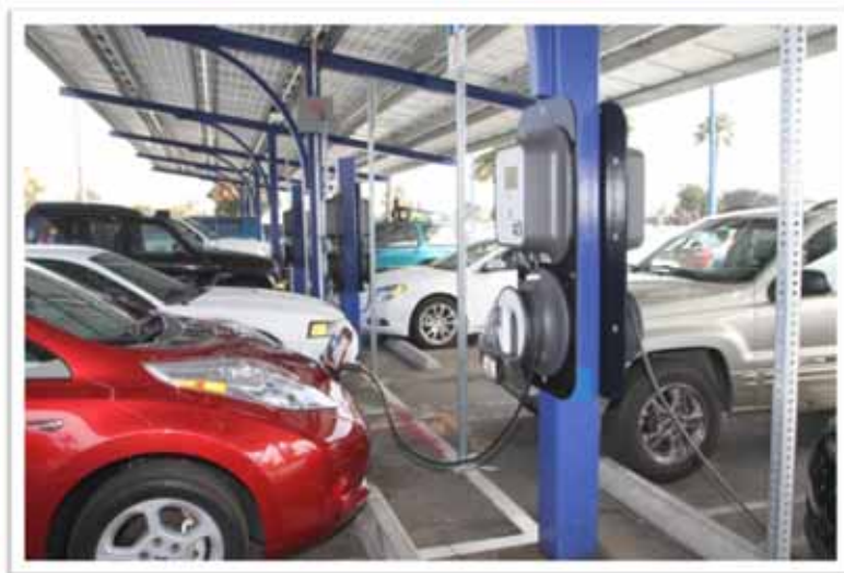
Wall-mounted EVSE installed in parking garage with overhead surface-mounted conduit
