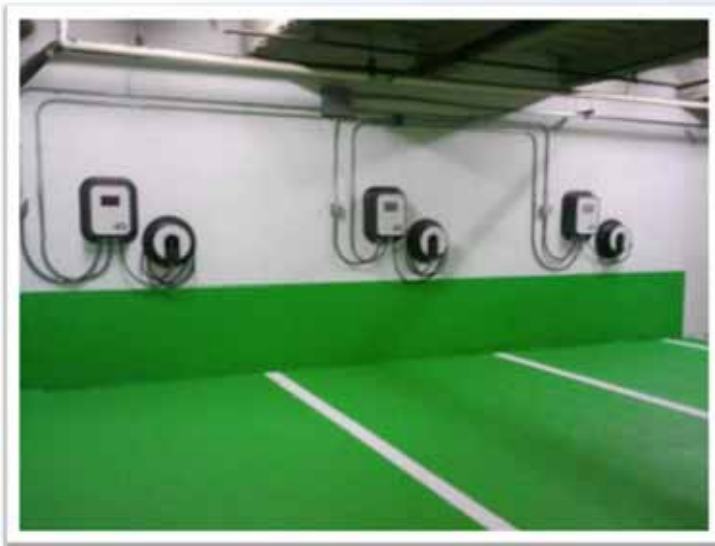
Wall-mounted EVSE installed in parking garage with overhead surface-mounted conduit
