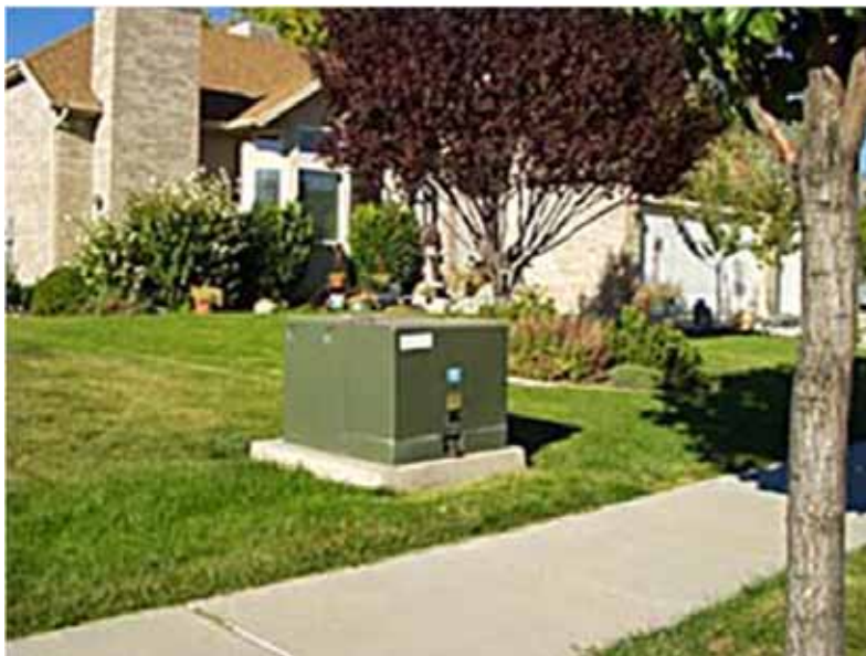
Figure 11-55. Pad-mounted residential distribution transformer [24].
