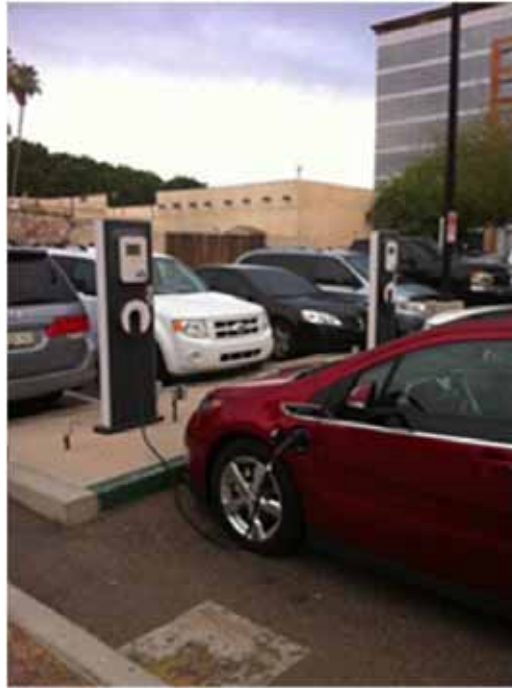
Figure 11-96. AC Level 2 EVSE charging station at Monti's la Casa Vieja in Tempe, Arizona.
