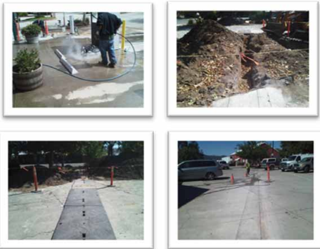
Figure 11-5. Examples of trenching for DCFC electrical conduit and wiring.
