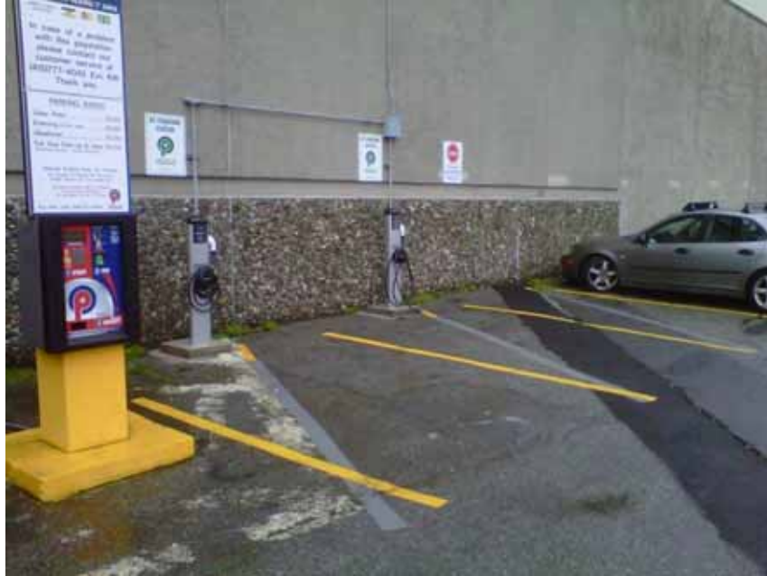
Figure 6-3. ChargePoint EVSE installation in the San Francisco area.
