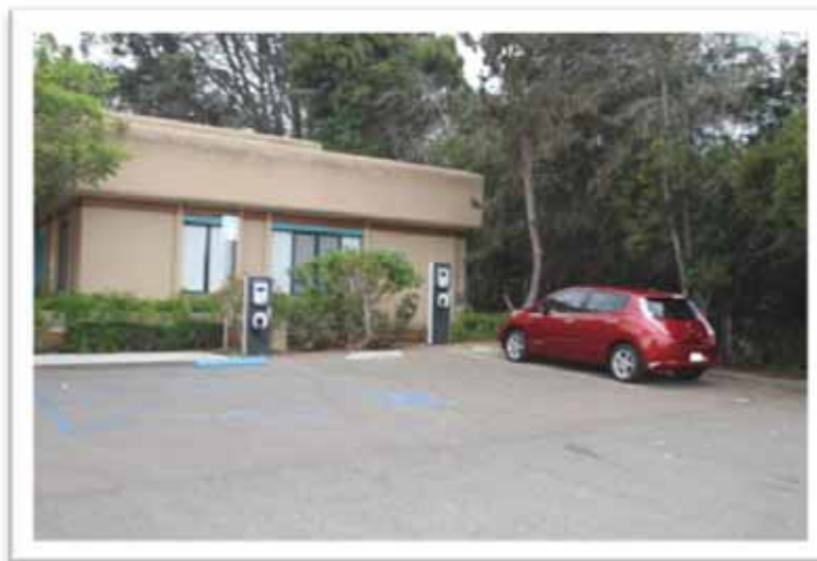
Figure 11-95. Americans with Disability Act -access compliant EVSE installation.
