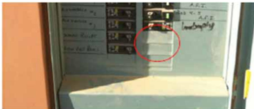
Figure 11-27. Circuit breaker panel and space for two circuit breakers to support AC Level 2 EVSE.
