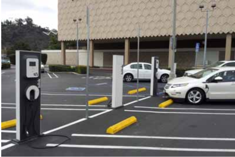
Figure 9-25. Multiple EV Project AC Level 2 EVSE installed at a department store parking lot.
