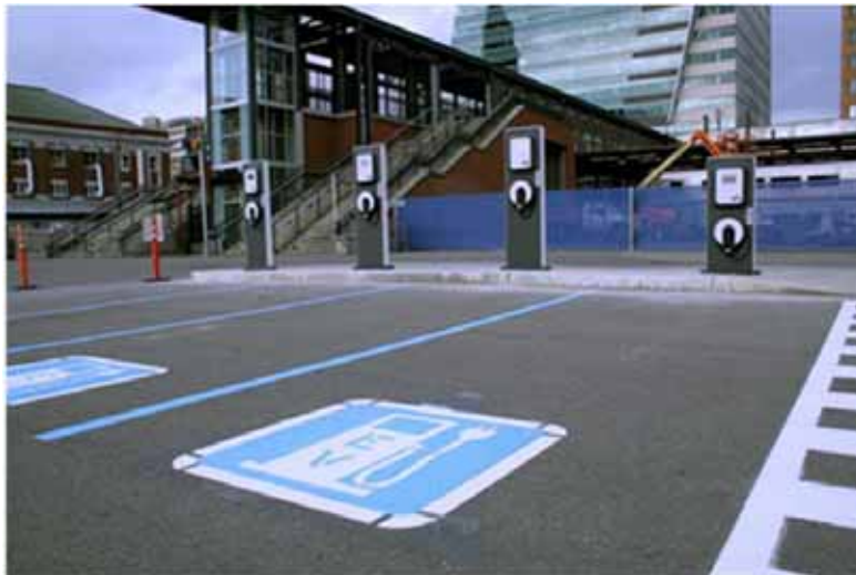
Figure 11-123. EV parking stall with recommended symbol on pavement.
