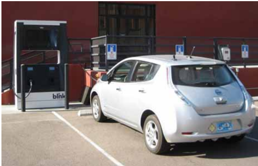
Figure 9-6. EV Project DCFC installation in the Phoenix, Arizona area. The DCFC is charging a Nissan Leaf.
