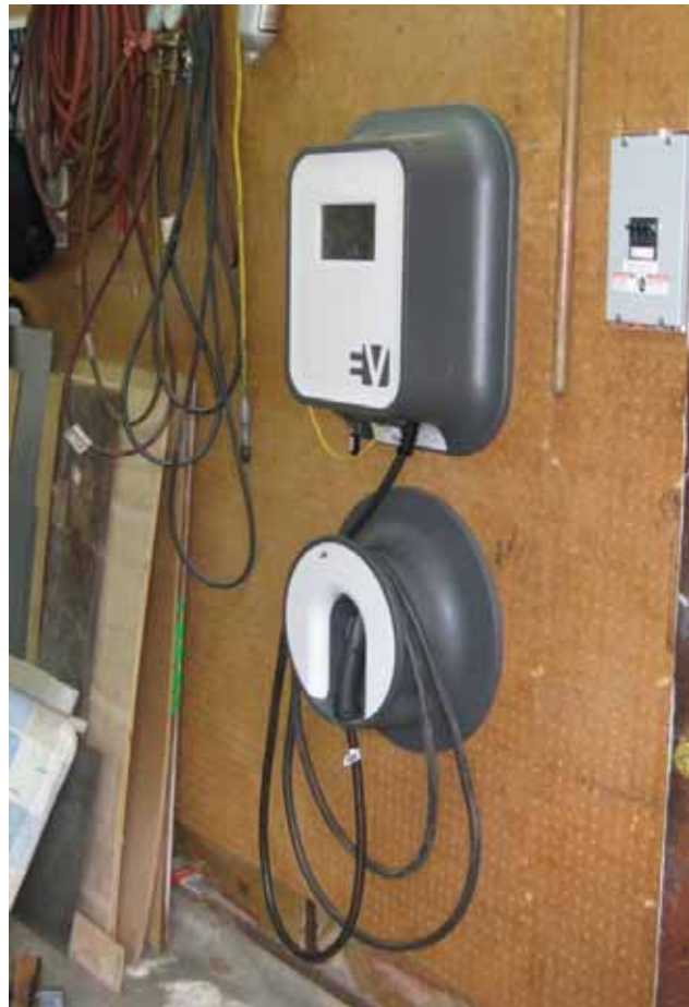
Figure 9-1. EV Project residential EVSE hung on a residential garage wall.
