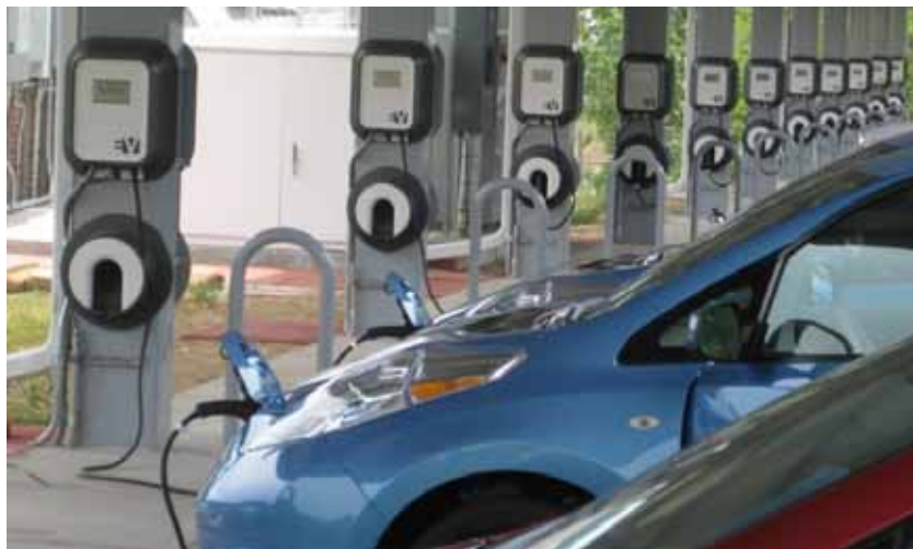
Figure 9-4. EV Project commercial EVSE installation in the Oak Ridge, Tennessee area.
