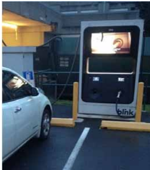
Figure 11-2. Dual-port Blink DCFC (photo courtesy of Plugshare.com).
