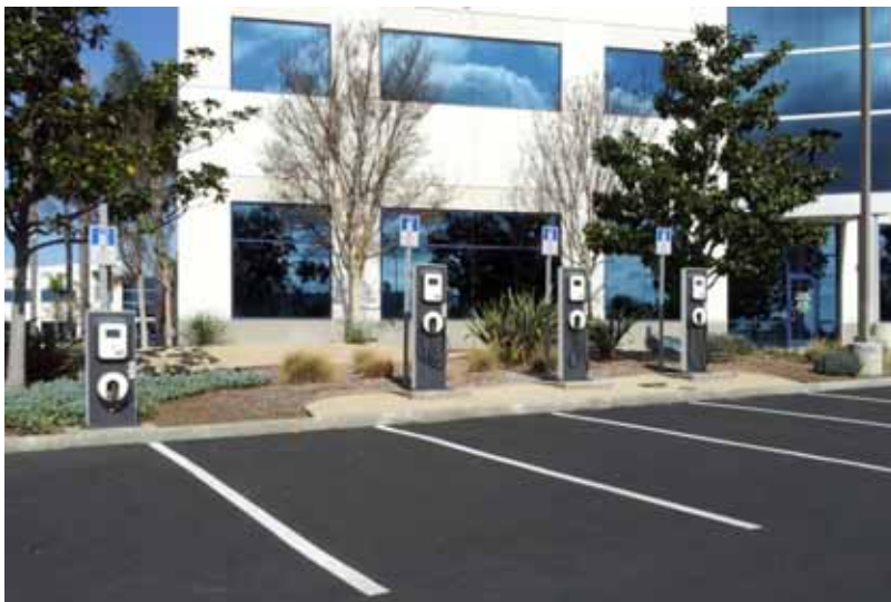
Figure 9-27. Multiple EV Project AC Level 2 EVSE installed at an office building parking lot.
