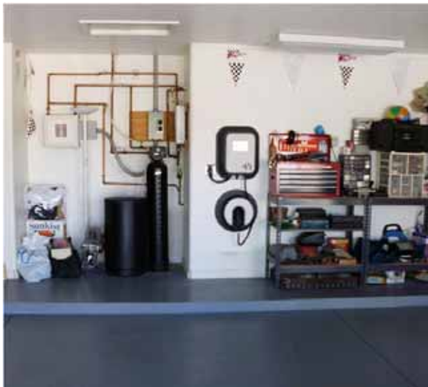
Figure 11-28. Clear floor and wall access to Blink EVSE.
