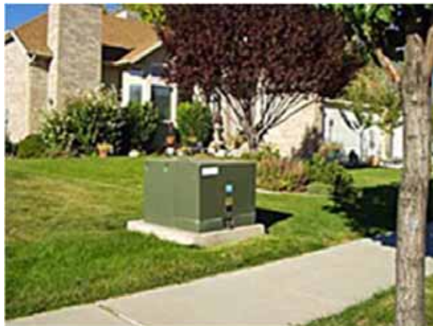
Figure 11-71. Pad-mounted residential distribution transformer [31].
