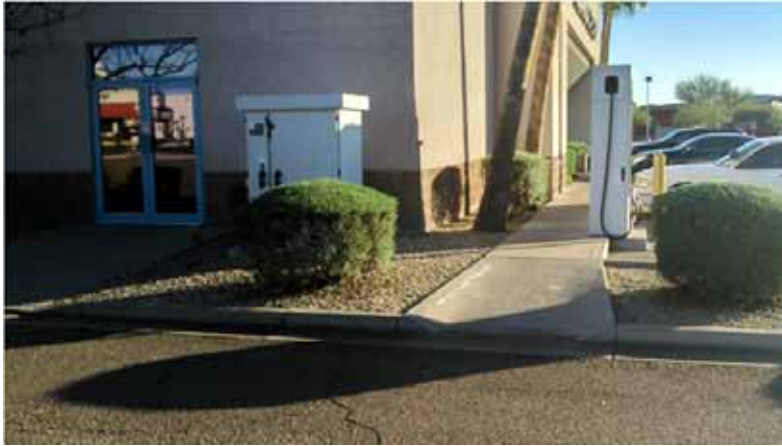
Figure 11-1. GPU (left) and CDU (right) for Blink DCFC.
