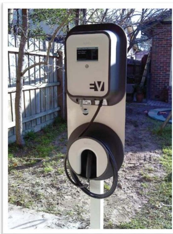
Figure A12. Wall-mount EVSE installed on a post with backing plate. Conduit installation trenched and recovered with soil like pedestal.
