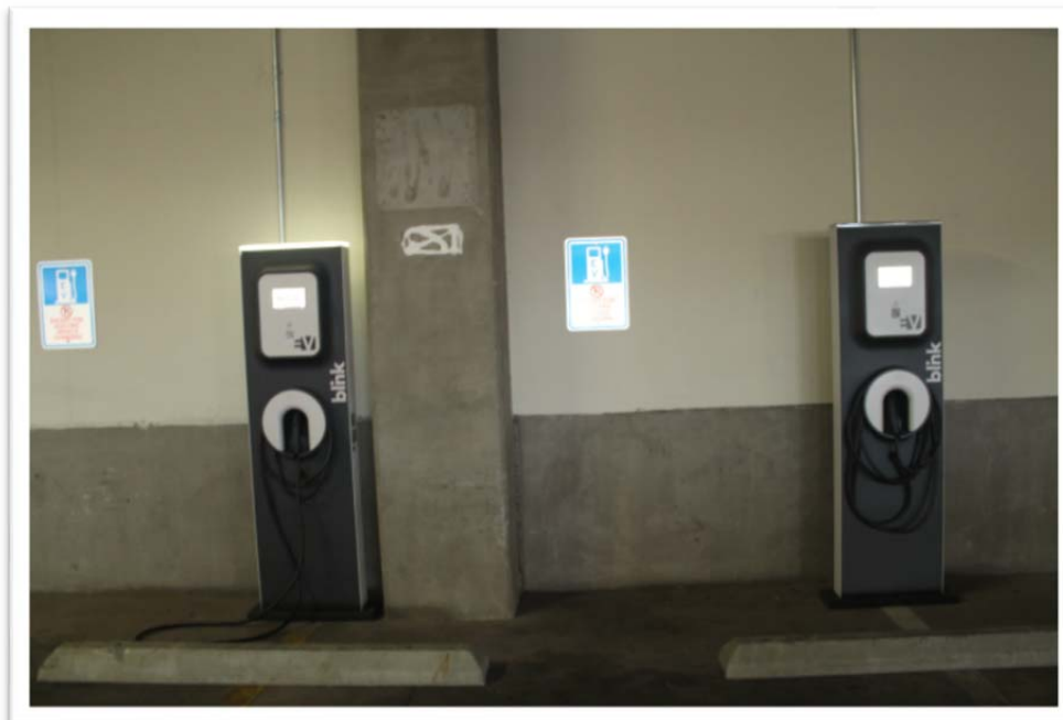
Figure A10. Pedestal EVSE installed in parking garage with overhead surface-mounted conduit.
