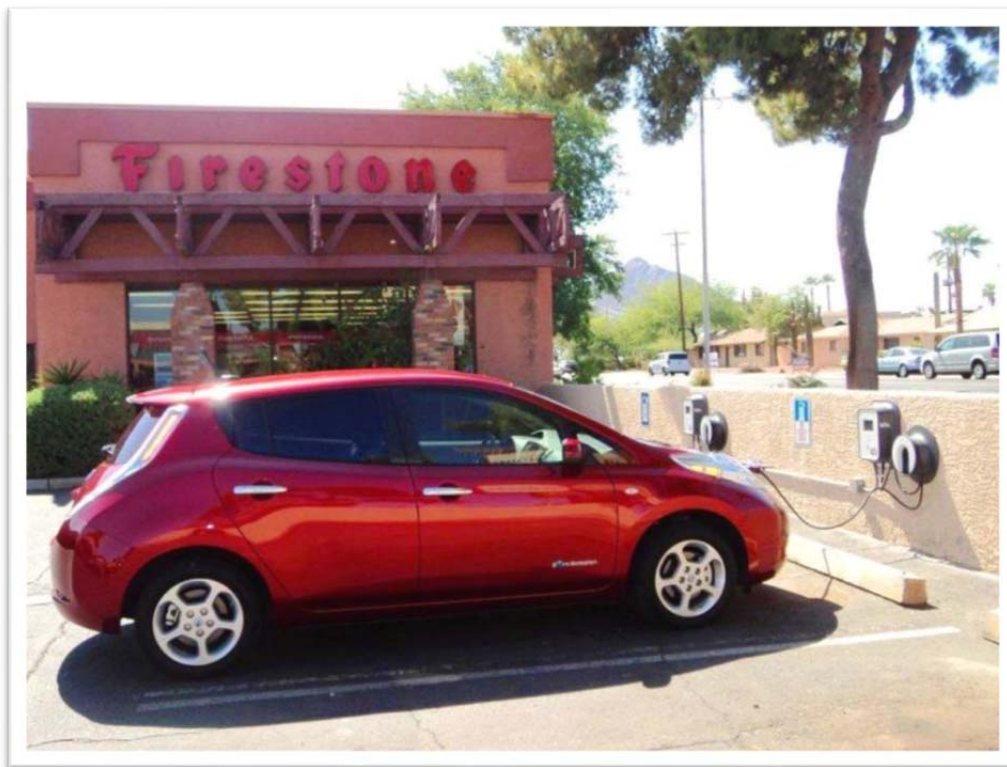
Figure A9. Wall-mounted EVSE installed on block divider wall with surface mounted conduit.
