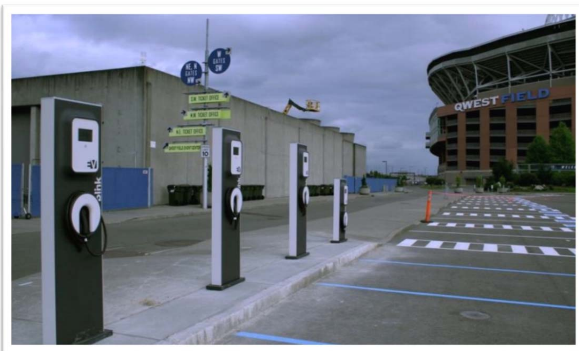
Figure A5. Pedestal EVSE installed on concrete sidewalk, requiring breaking out and re-pouring concrete for underground conduit.
