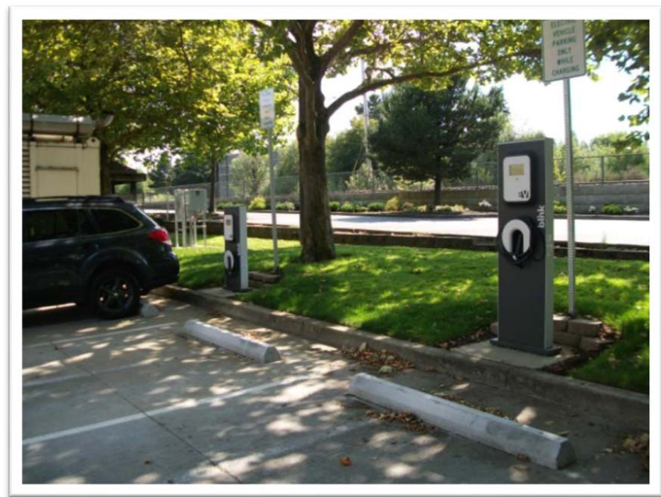
Figure A2. Pedestal EVSE installed on concrete pad, with underground boring for conduit.
