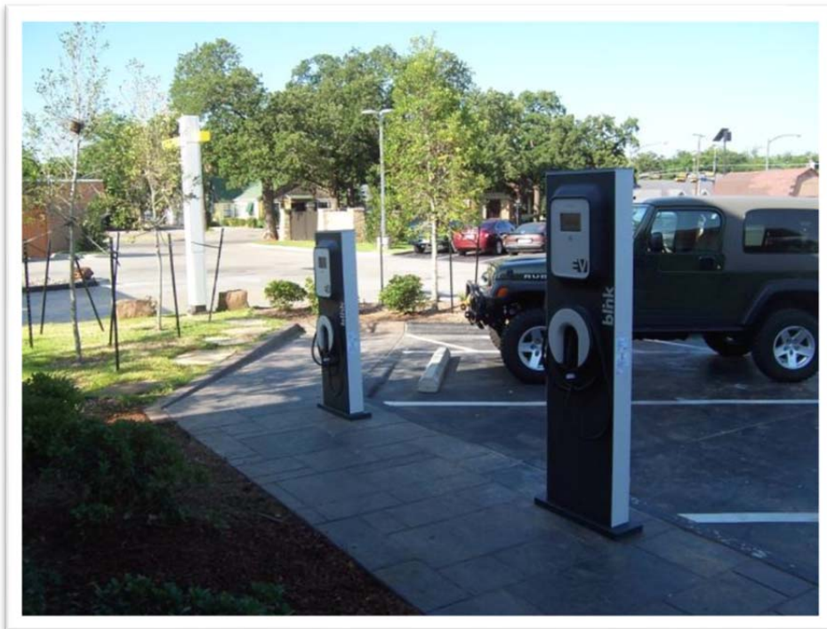
Figure A1. Pedestal EVSE installed on decorative paving; removal and replacement required for underground conduit.
