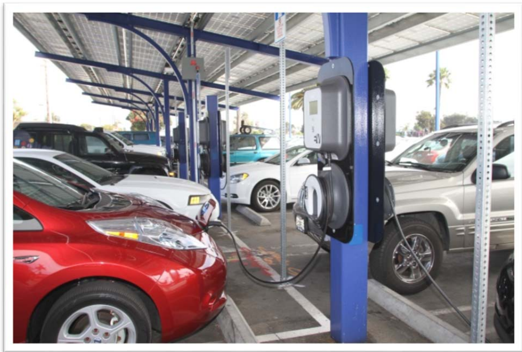
Figure A7. Wall-mount EVSE installed on building pillar with backing plate and overhead surface mounting for conduit.
