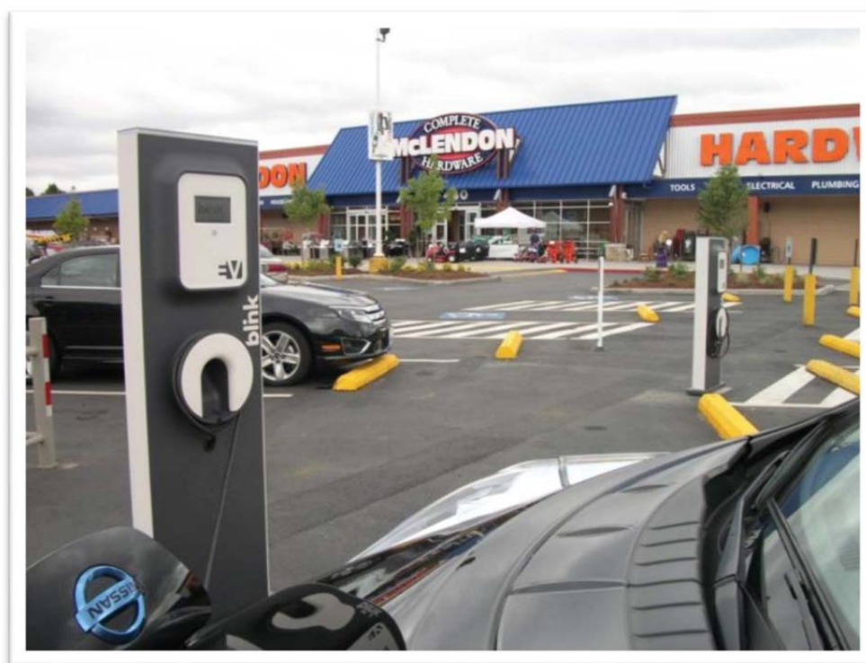
Figure A4. Pedestal EVSE installed on asphalt, with trenching and repaving for underground conduit.
