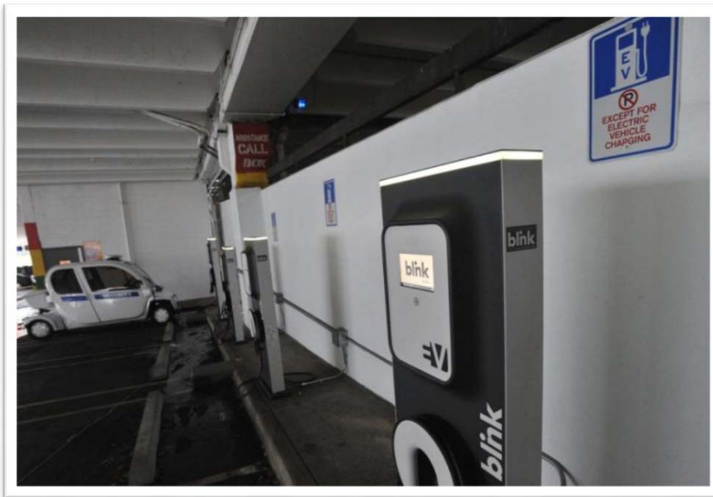
Figure A11. Pedestal EVSE installed in parking garage with wall-level, surface-mounted conduit.
