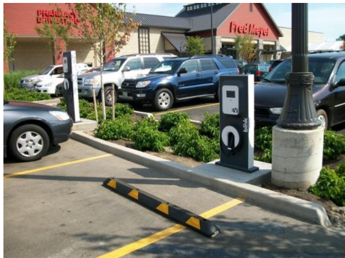
Figure 4. Publicly accessible AC Level 2 EVSE installed in a prominent location on the host's property.
