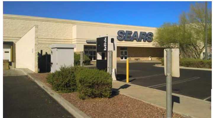
Figure 6. Example of one of the least expensive installations.
