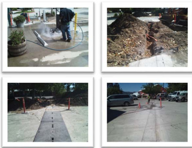
Figure 5. Trenching for DCFC electrical conduit and wiring.
