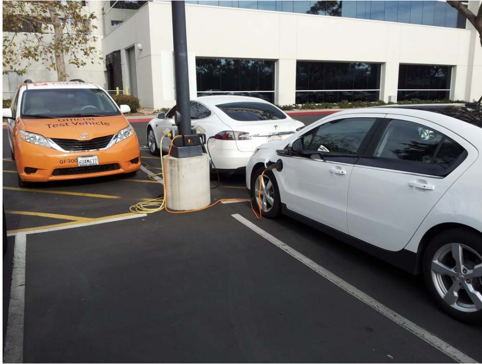
Figure 3. Multiple AC Level 1 in a parking lot at the base of a light pole.
